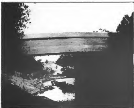
Patoka River, near Duff. Such Bridges were Raised to Permit Flat-boats to Pass Under Them.
